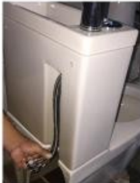
Step 4: Connect hot & cold water hose to the tap and connect the other end to outlet of the valves.
